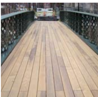
Yale Bridge deck using Greenheart construction
