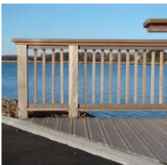
6x6 posts and at railing Newbury port 1 year weathered
